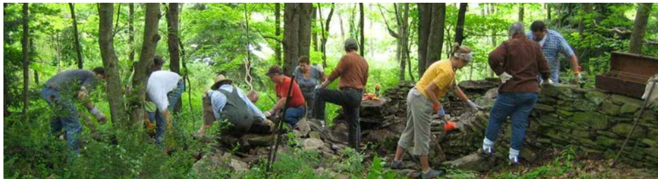
The rebuilding of a stone wall—beginning to end.
