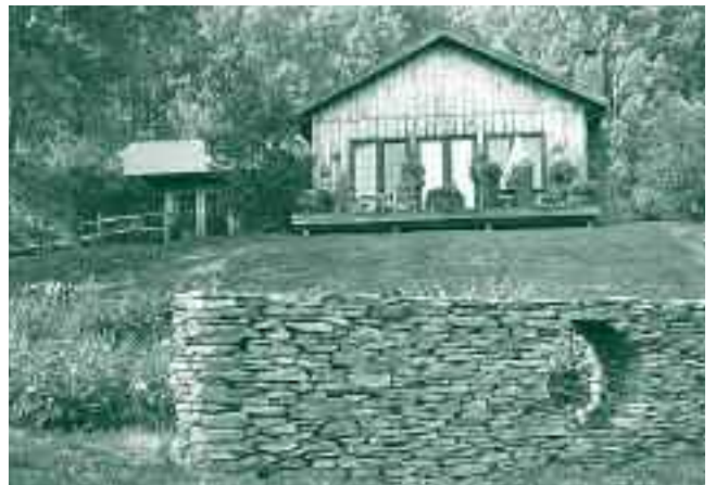
Unique stone wall at Kickback Farm
