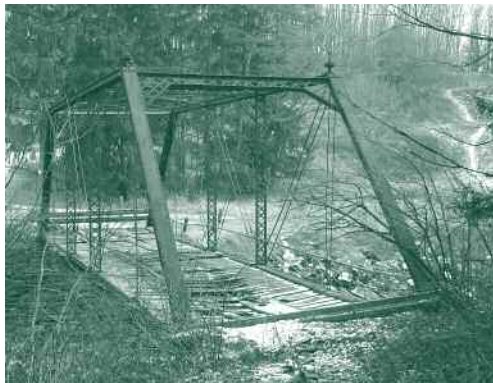
The existing 19th-century iron bridge
